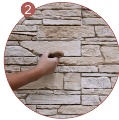
2 I remove any excess adhesive
