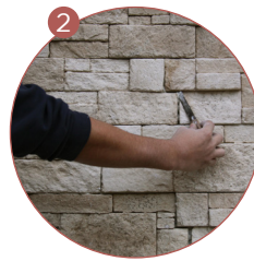
2 | remove any excess adhesive
